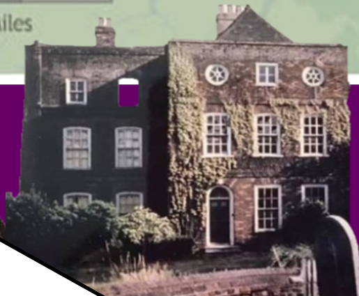
SWANSCOMBE MANOR HOUSE
